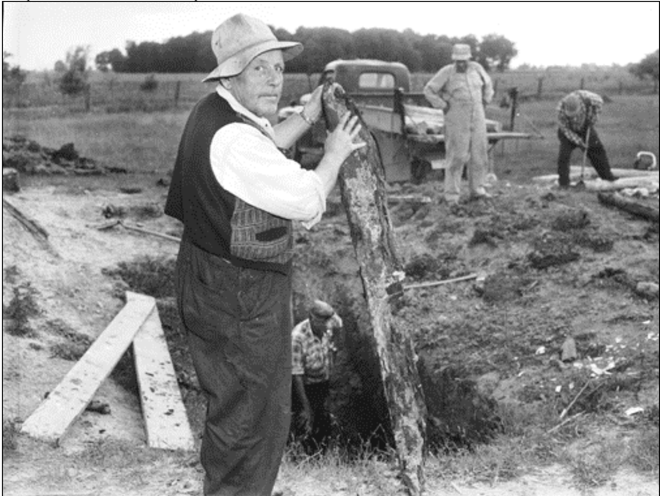
Figure 9. Angus Sutherland, foreman for Fairbank Oil Properties, in 1957, examines a plank for the cribbing of North America's first well to produce crude oil for the nascent petroleum refining industry (initially the coal oil refining industry). The well was dug in 1858 by workers employed by J.M. Williams. [Lambton County Museum, 365642-01].
